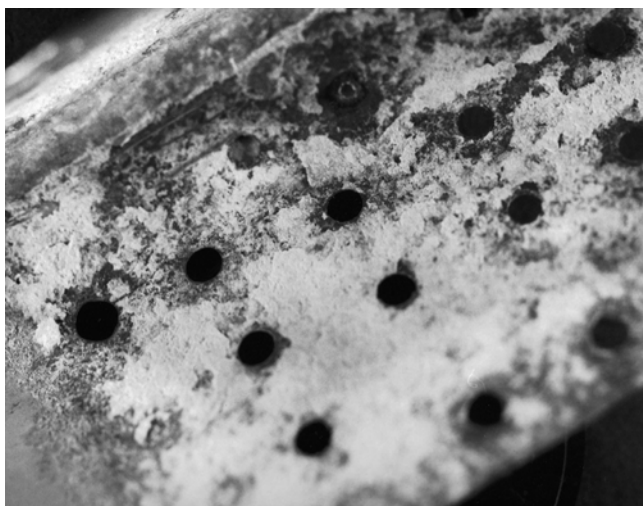
Figure 3-23. Aluminum Surface Corrosion Products
