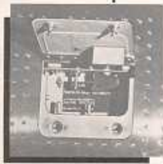
REFUELING PRECHECK SWITCH PANEL *
